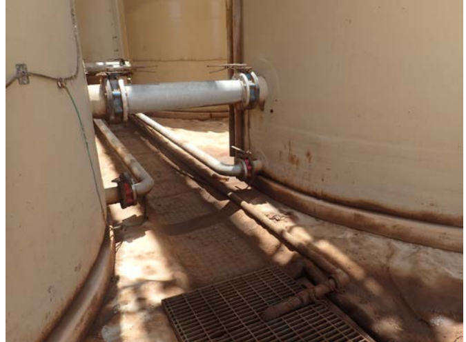
Fig. 8 - Tanks Bonded Together Design
