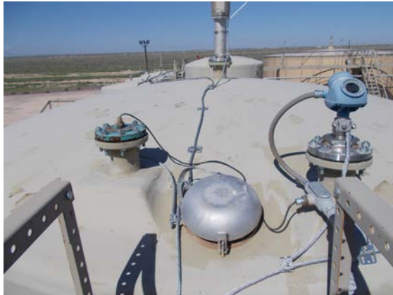
Fig. 6 - Tank Vessel Bonding Install
